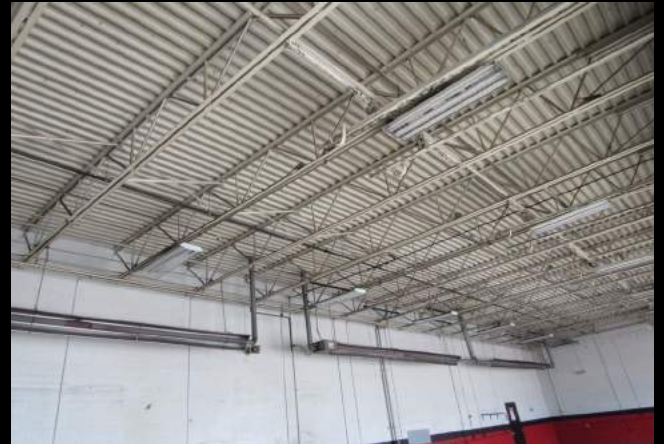
STEEL CEILING JOISTS AND RADIANT HEATERS
