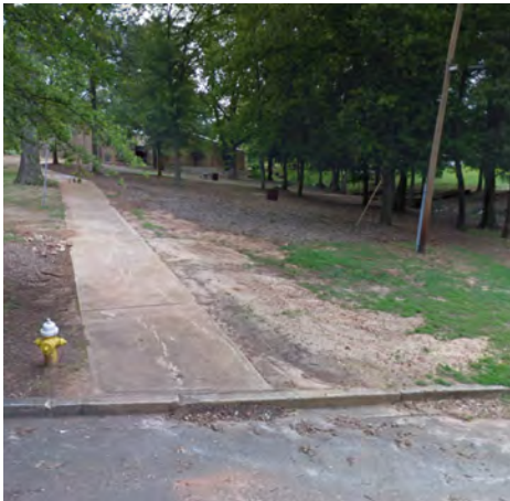
Curb cuts: Simply cutting this curb on Douthit Street would help increase access to the community center for parents with strollers, wheel chairs, cyclists, roller skaters and others with wheels
