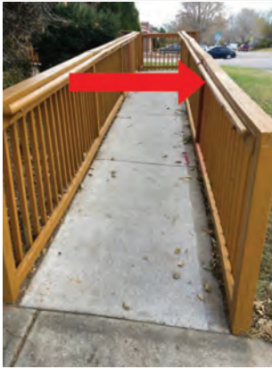
Front service ramp. Handrail is loose
