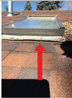
Skylight flashing is separated from roof
