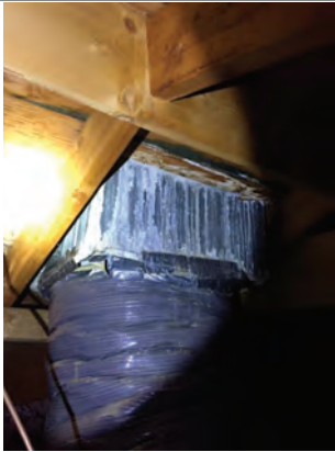
Evidence of leaking flashing around evaporative cooler.
