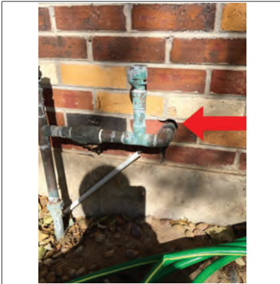
Caulk as needed around wall penetrations
