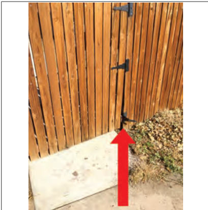
East gate hinge is damaged/loose
