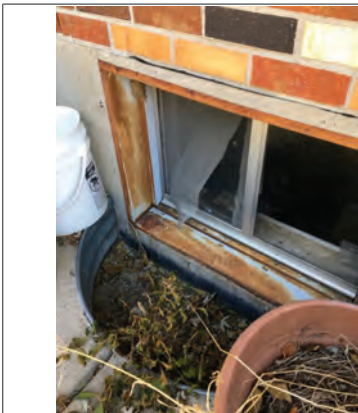
Damaged basement screen window
