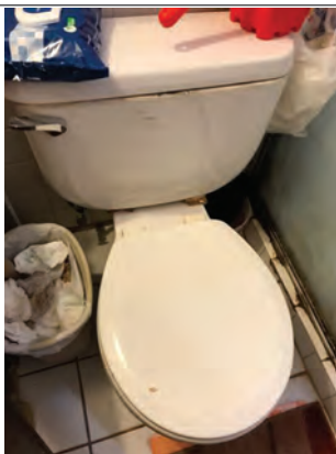
Tank is wedged for support
