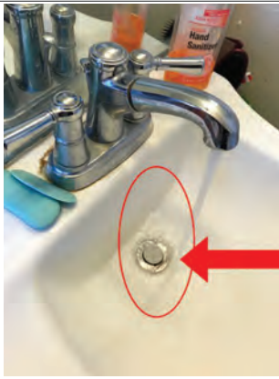
Sink stopper does not stay closed
