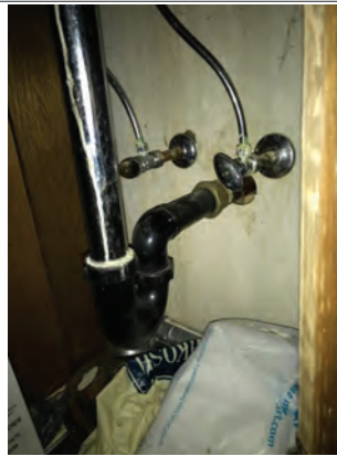
Corroded valves at sink
