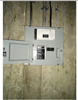
Basement sub panel. Breakers have mechanical locks in place to keep them from tripping. Unsure if this is a safety concern or if licensed electrician installed them and breaker in main panel is responsible for wire protection. Recommend electrical inquiry be made.
