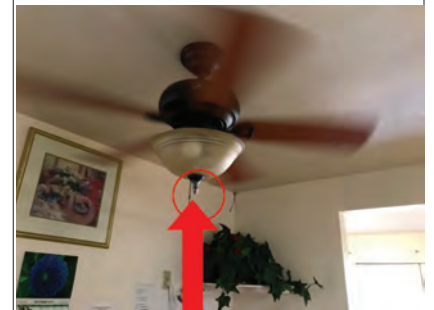
Screw does not hold globe in place, tape is being used Fan speeds are not able to be changed
