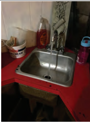
Only hot water is available at wet bar sink. Right handle or cold water does not turn.
