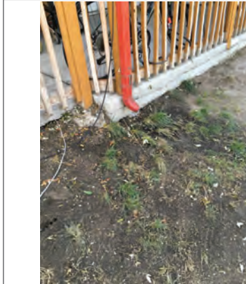
Missing downspout extension
