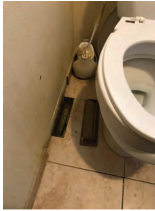
Heater vent register loose
