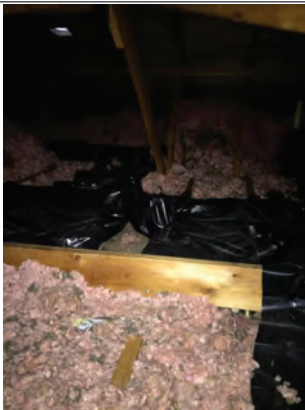
Displaced insulation
