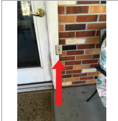
Patio GFCI receptacle would not trip when tested
