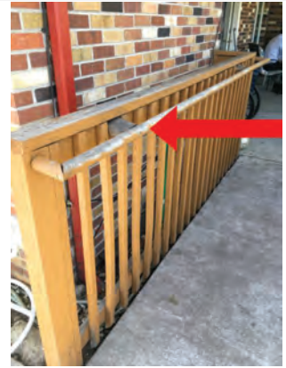
Handrail is loose
