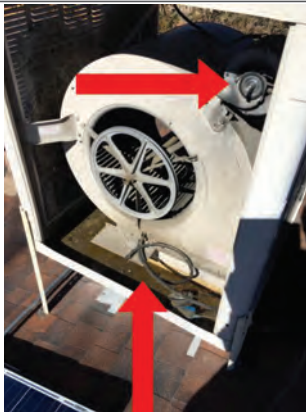
Broken belt and sheave has fallen off motor.
