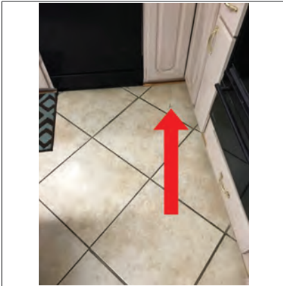
Kitchen floor Cracked tile
