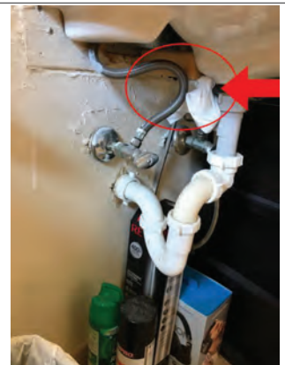
Questionable stability and leak free sink There appears to be a board wedged for support of sink Uncertain why paper towel is wedged in place.
