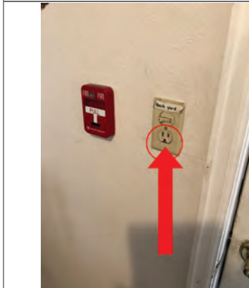
Dining room Damaged receptacle
