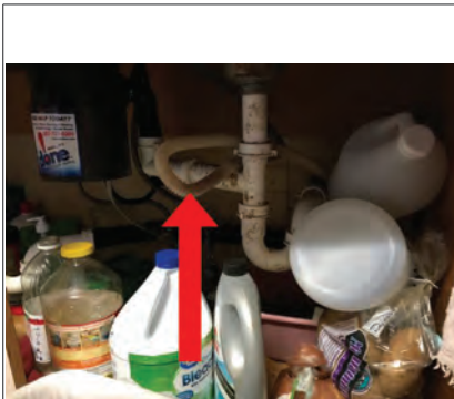
Plumbing under kitchen sink No high loop
