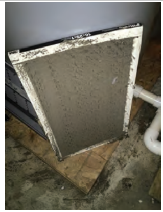
Severely dirt covered furnace filter. Filter was intentionally left out of furnace for obvious reasons.
