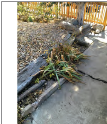
Deteriorating retaining wall
