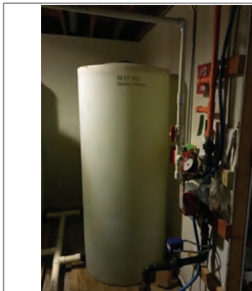
Fire suppression system water tanks
