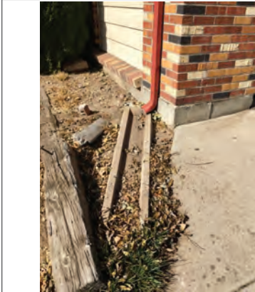
Splash block may not channel water effectively
