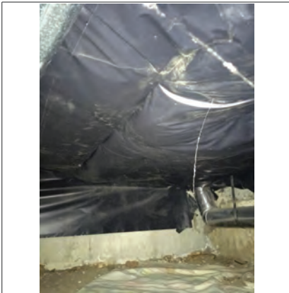
Vapor barrier installed over floor joists in crawlspace
