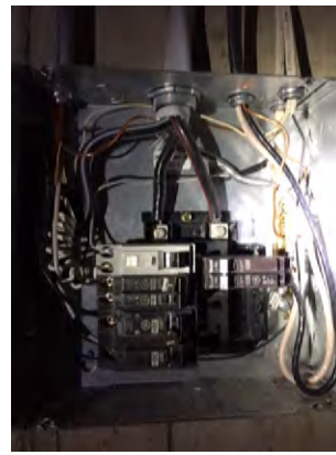
Basement sub panel. Cover removed for inspection.
