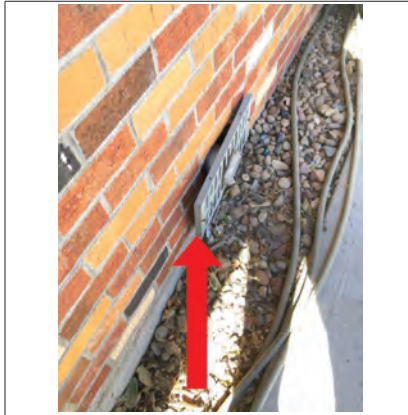
Loose crawlspace vent
