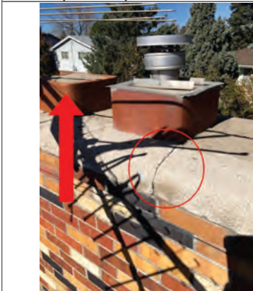
Chimney cap has cracks. Note concrete sealed flue liner
