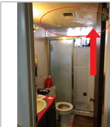
Bathroom 3 in basement Water damage on ceiling evidenced by peeling paint
