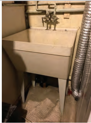
Inoperable laundry sink faucet Unable to determine usefulness. Not evaluated Faucet handle missing
