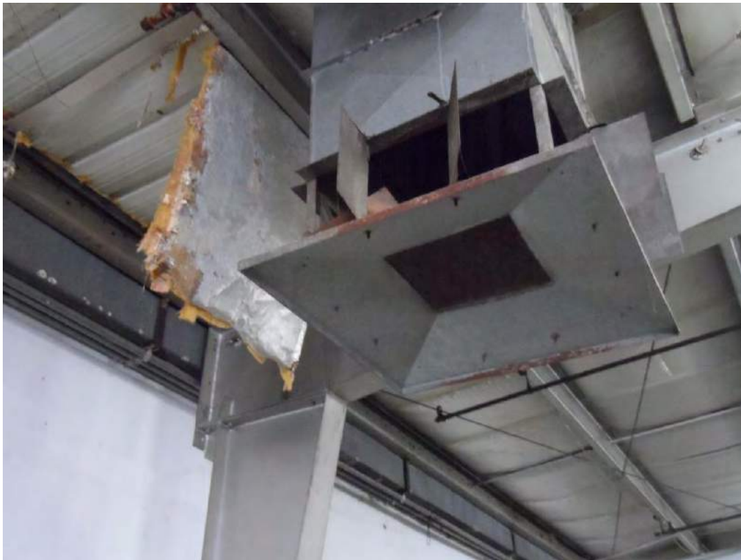
11. View of insulation falling from the ceiling inside the proposed bus maintenance shop.
