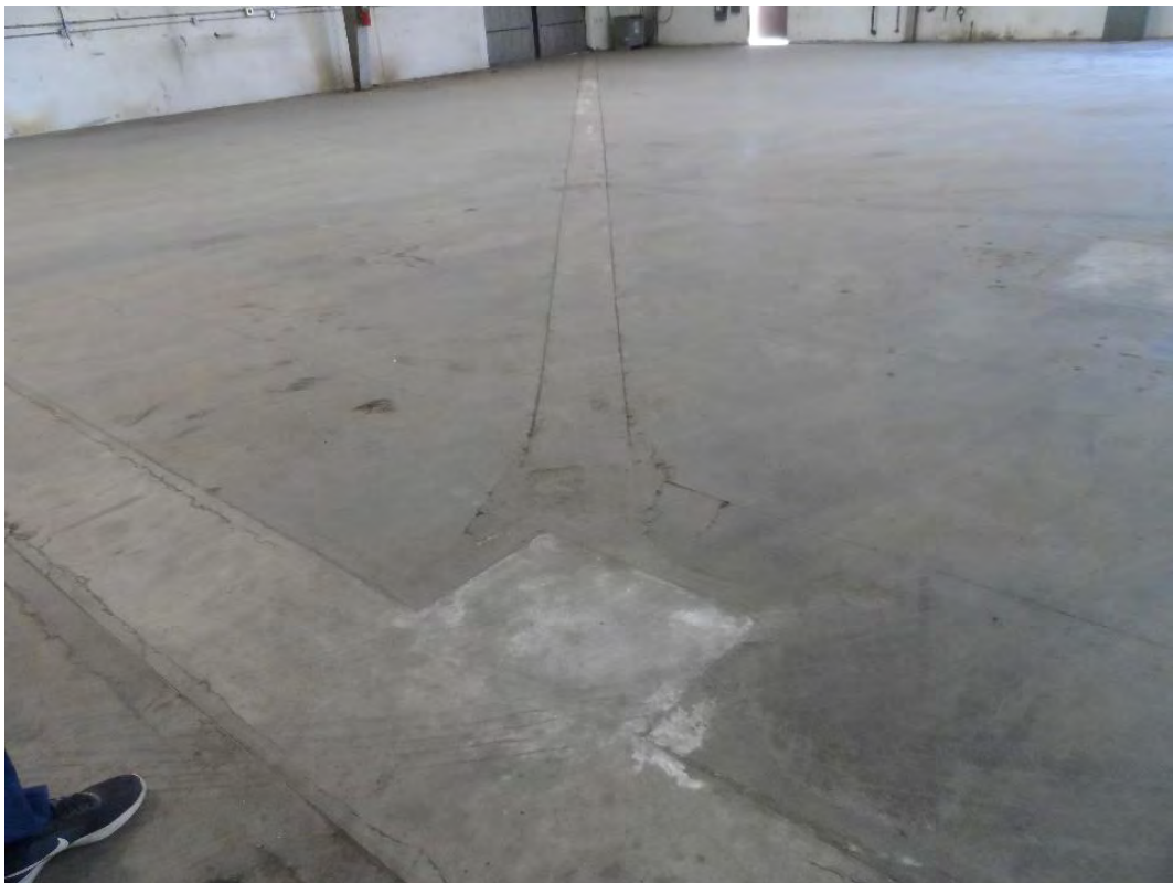
12. View of cuts in the concrete floor of the proposed bus maintenance shop.
