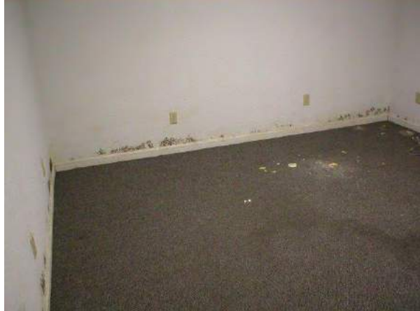
Visible mold along baseboard of offices of vacant space formerly occupied by Kroy Industries.
