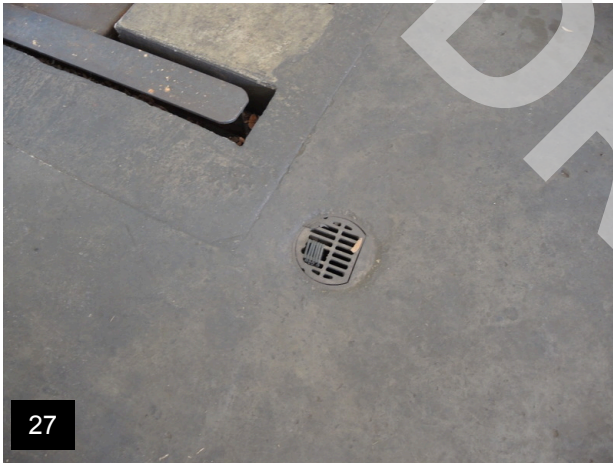
27 Floor drain in car repair area
