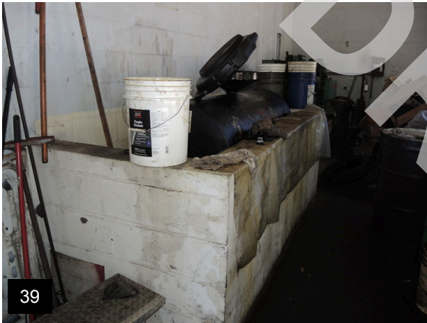
39 Spill containment enclosure and 300-gallon waste oil AST
