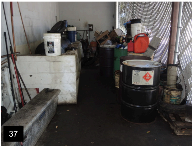
37 Drum storage area with heavily stained floor
