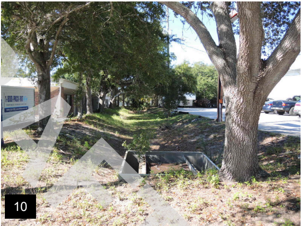
10 Storm drain and stormwater swale
