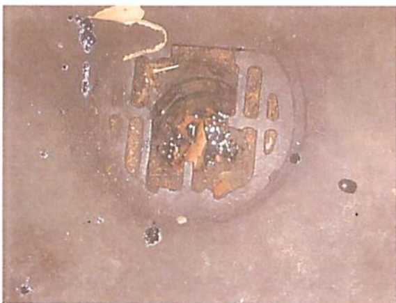
Photo ID # IMG_0769 /10:45 AM – Oil in floor drain (same as above)
