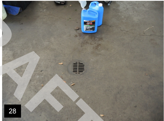
28 Floor drain in car repair area
