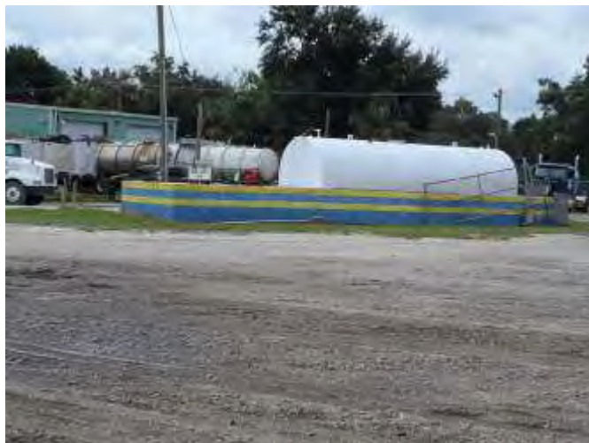
8. Diesel Fuel 10,000-gallon AST
