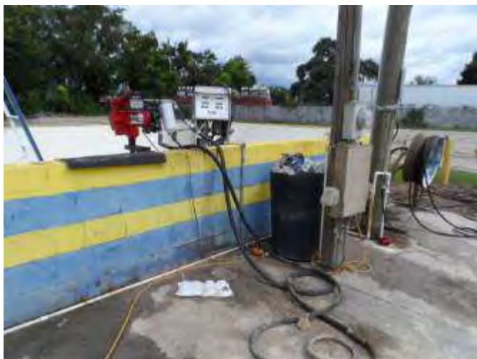
9. Dispenser for 10,000-gallon diesel fuel AST
