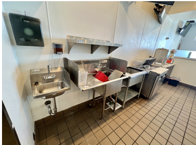
Sink #1 with hand washing station and floor drain
