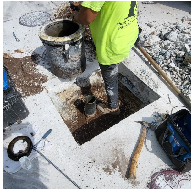
Diesel Spill Bucket Removed For Riser Repair
