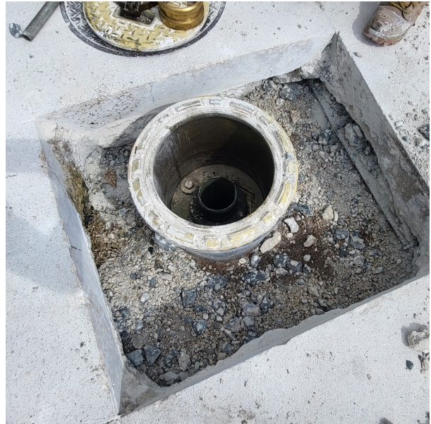
Diesel Spill Bucket Excavation
