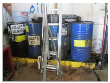
45. View of waste oil drums in secondary containment in the automotive tenant repair space on Parcel 2.
