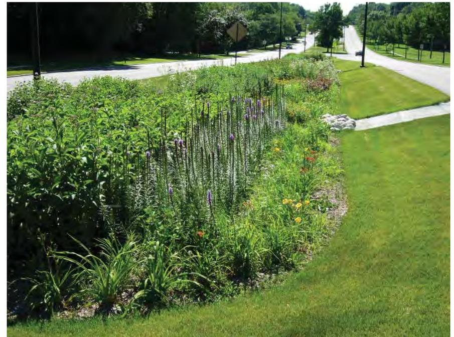
Figure 8.8: Bioswales alongside the road and in the median
