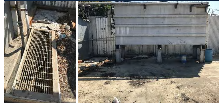
Stormwater Filtration System
