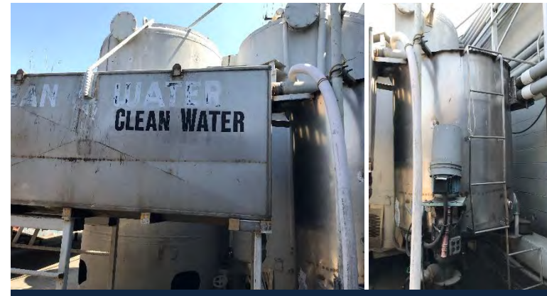
Stormwater Filtration System
